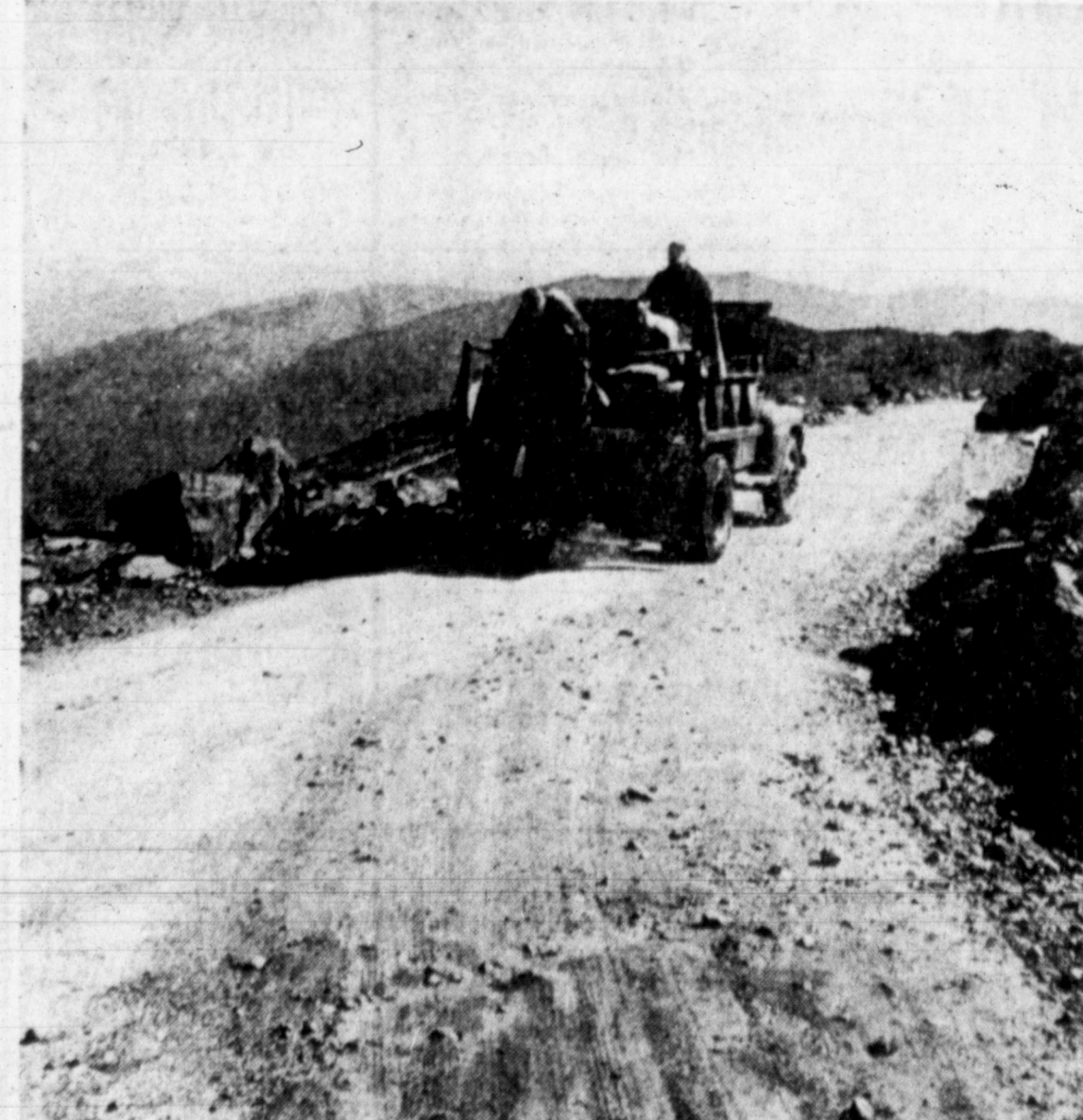
DUST BITES DUST —Workmen powder the dust on Mount Washington road near Gorham, N. H., to prevent the road from being blown away by hurricane-force winds that lash the 6,288-foot mountain giant. The Solvay calcium chloride flakes draw moisture from the atmosphere which helps control the dust and makes the surface of the road compact.
