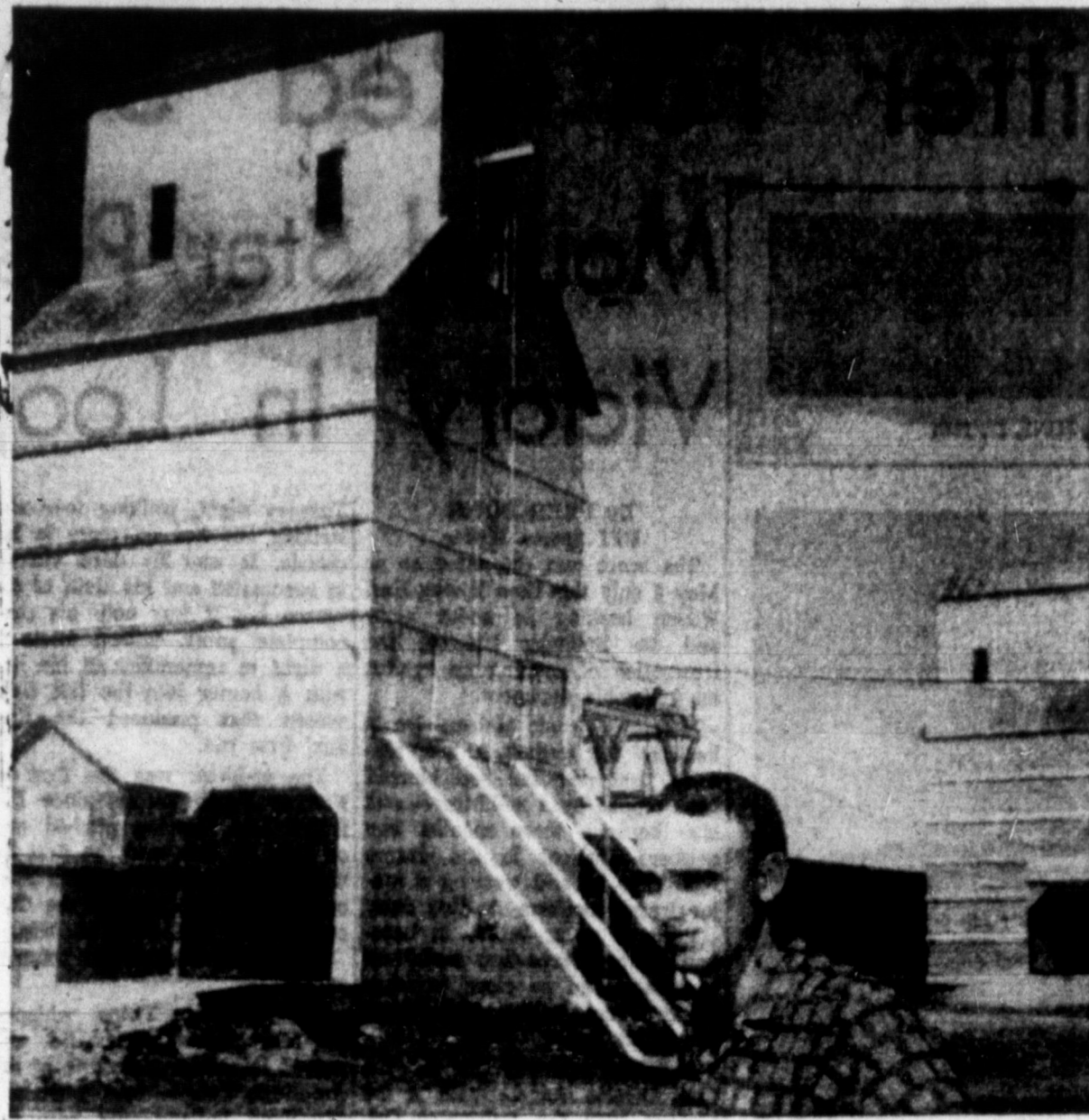
NEW MANAGEMENT — Jack Villines, manager of the Pampa branch of the Trans Con Elevators, Inc., Heaton Switch, stands before the two elevators while waiting for the last of the wheat harvest trucks to come in. Formerly owned by Laketon Wheat Growers Association, the elevator is under new management and has taken in 25,000 bushels of wheat since it reopened June 1. Located nine miles east of city on the Wheeler highway, the elevator will stock anhydrous ammonia and dry bulk fertilizer and weed and insect killers for area farmers. (Daily News Photo)
