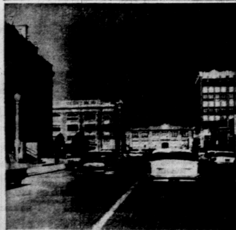
DOWNTOWN PAMPA —This is a street in the downtown area that shows a portion of Pampa's mall of public buildings. At left front is the City Hall. Left center is the Gray County Courthouse. Directly at the end of the street in the distance is Pampa Junior High school. On the right is the Combs-Worley office building.
