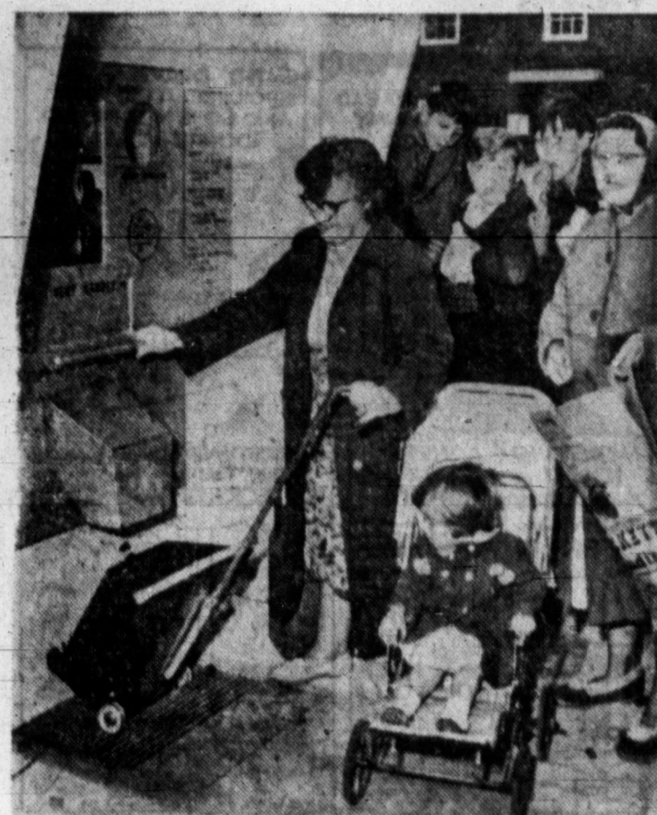
'FUELY' AUTOMATIC —Britain's first automatic coal-feeding machine wins the hearty approval of the housewives in London. The machine, a coin-operated electronic device, holds six tons of coal and dispenses it loosely.
