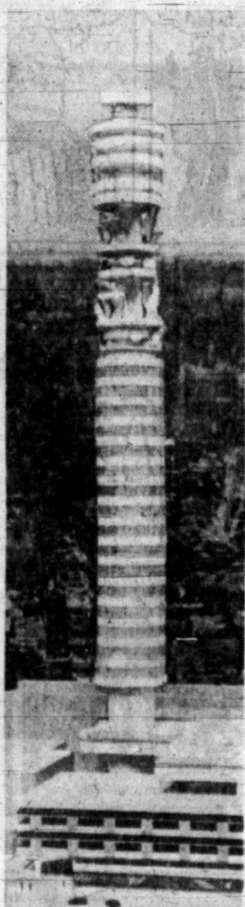
TALLER THAN —This model shows a building which will be a reported 603 feet high, taller than any other in Britain. The signal transmitting and receiving tower will also contain a revolving restaurant that will give diners a panoramic view of London.
