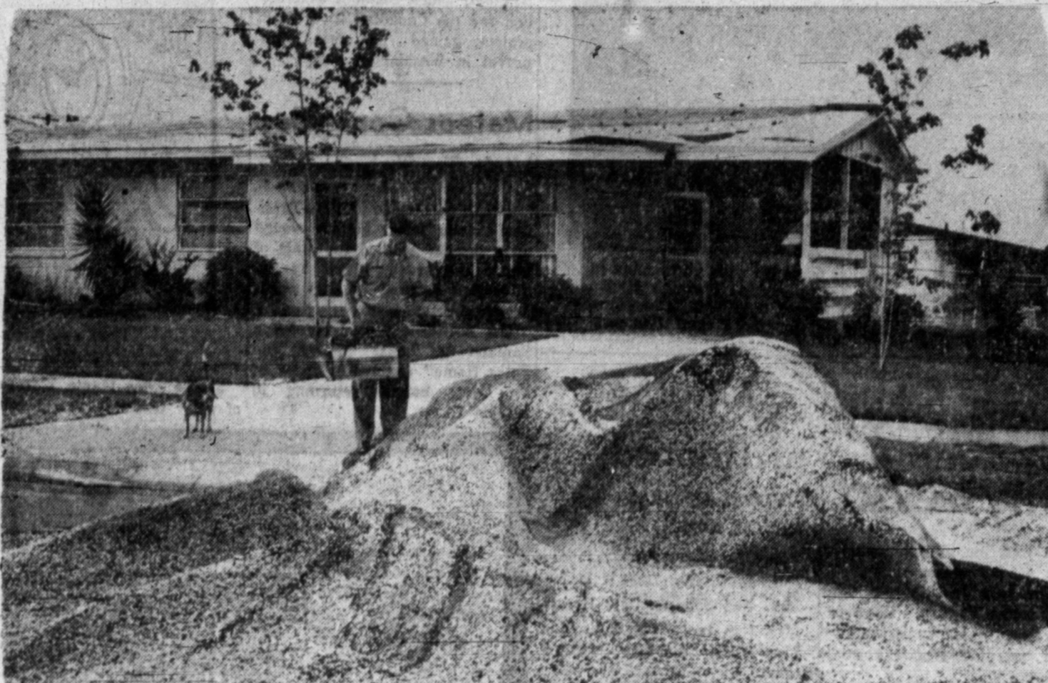
GONE WITH THE WIND —Feeling strange without a roof over his head, Tom Murray, of Jacksonville, Fla., picks up his mail box after a furious windstorm ripped off his roof and deposited it on his front lawn. Rain, flood and wind damaged Murray's home was estimated at $4,000. If he leaves the roof there, he will have the beginnings of an underground shelter and a leaking roof on his house.
