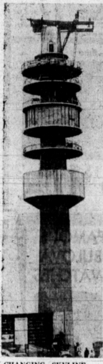
CHANGING SKYLINE —When completed, the Tryvanns Tower will be the highest point in the Oslo, Norway, area, about 1,960 feet above sea level. The structure itself, standing 360 feet tall, will be a radio tower primarily. It will also house a restaurant and a souvenir shop for visitors to the tall landmark.
