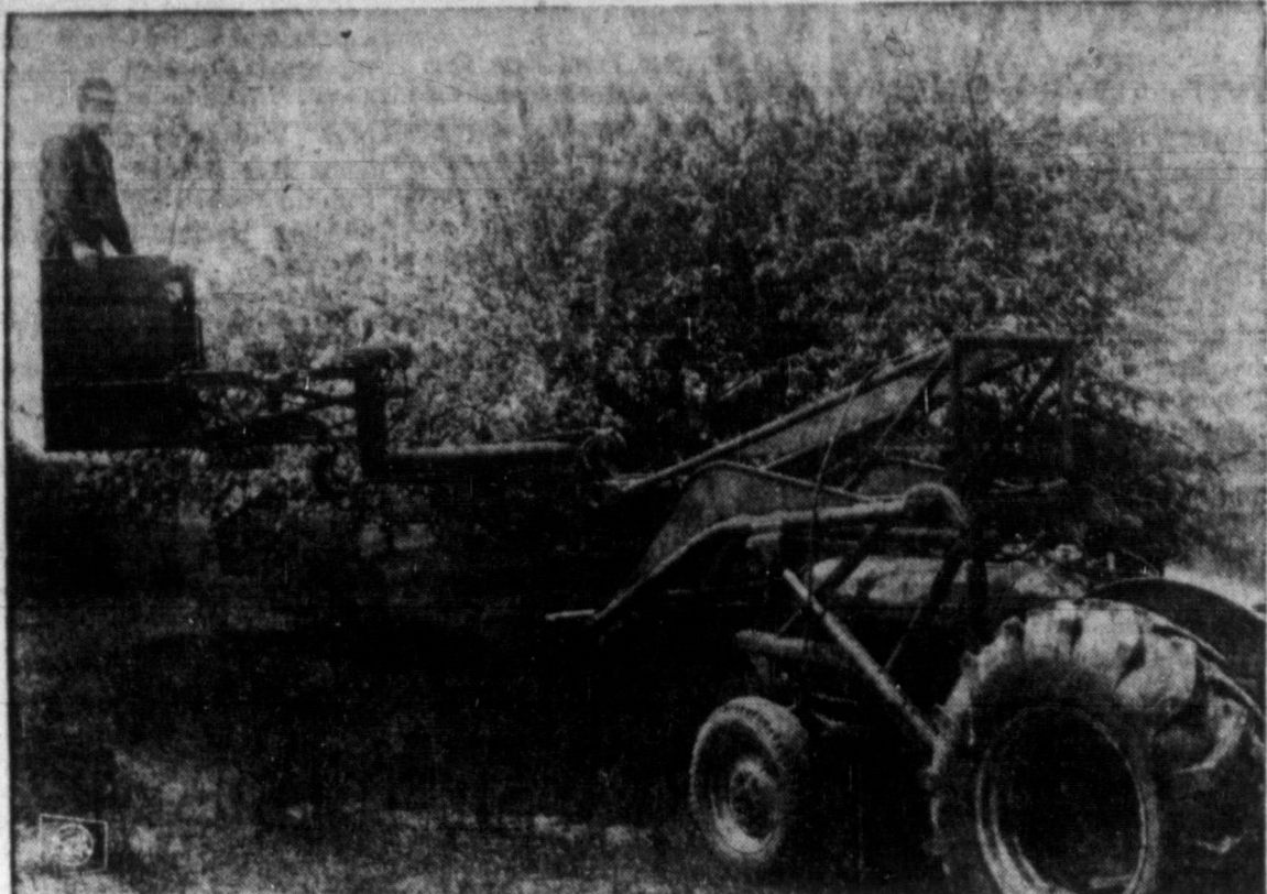
PRUNES COSTS TOO—Experimental "space basket," developed by the U.S. Department of Agriculture and the Michigan Agricultural Experiment Station, to cut the labor costs of pruning fruit trees, is tested at Lansing, Mich. One man drives the device while another manipulates levers which move him up (as high as 13 feet), down and sideways.
