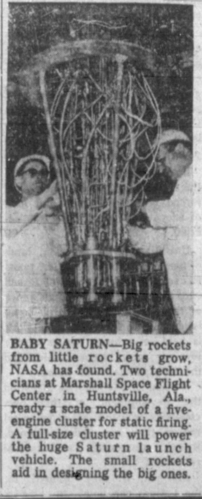
BABY SATURN—Big rockets from little rockets grow. NASA has found. Two technicians at Marshall Space Flight Center in Huntsville, Ala., ready a scale model of a five-engine cluster for static firing. A full-size cluster will power the huge Saturn launch vehicle. The small rockets aid in designing the big ones.
