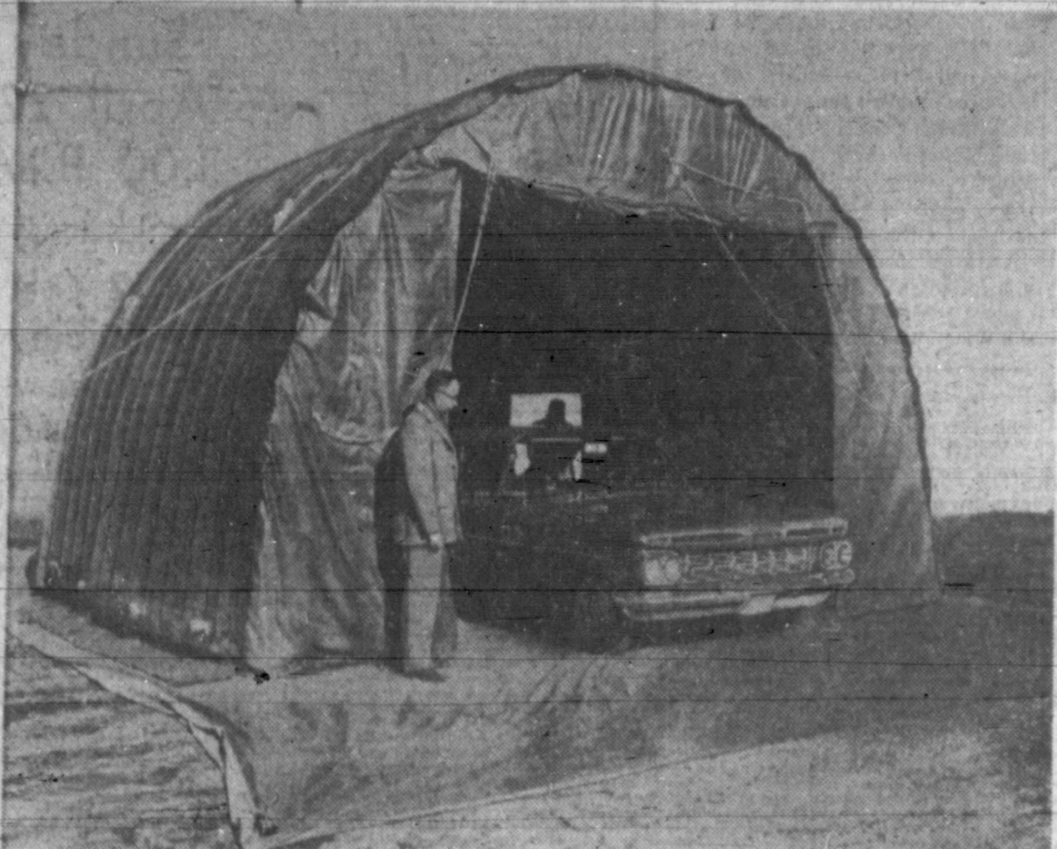
DO-IT-YOURSELF IGLOO —An inflatable shelter serves as a portable repair shop for the Quartermaster Corps in the polar regions. The shelter temporarily houses ailing trucks and tanks which are disabled on the move. The 20-foot-wide building can be inflated by a blower system in five minutes from a six by four foot portable package.
