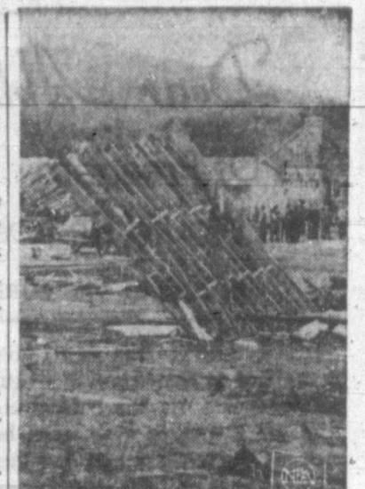
TORNADIC FILEDRIVER — These rafters from a wrecked building were driven four feet into the ground by a tornado striking Berwick, Pa.
