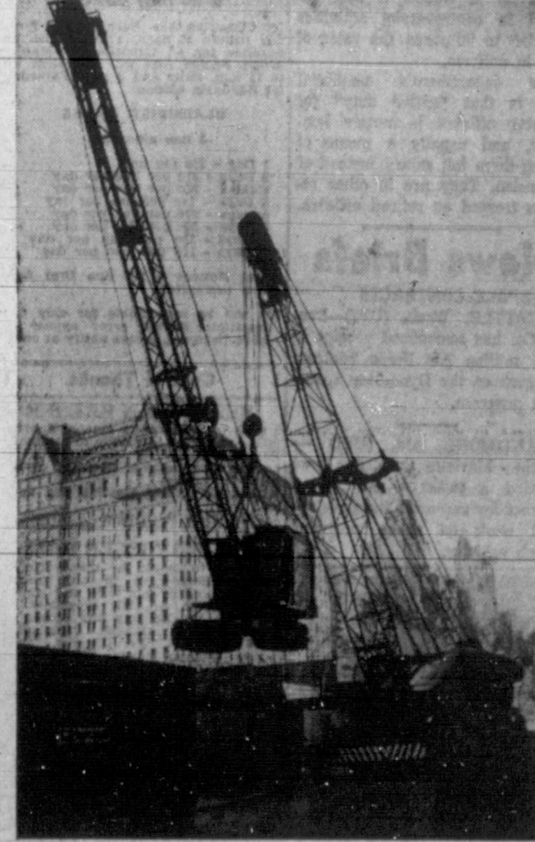
HITCH-HIKER —Resembling a cat grabbing its kitten by the scruff of the neck, this huge crane in New York lifts a smaller crane into position to do some lifting of its own. The little crane went up and over with nary a whimper.
