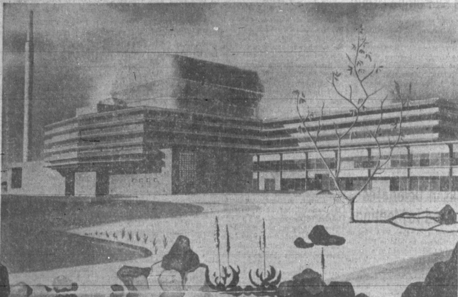
ATOMIC REACTOR FOR AFRICA —This artist's conception of the first nuclear research center in the Republic of South Africa will soon be solid reality as the construction gets underway. The light-water research and test reactor to be installed there was designed by Allis-Chalmers and South Africa's Energy Board. It will operate initially at 6,667 kilowatts (thermal), but is designed to operate ultimately at power levels as high as 20,000 kilowatts (thermal).
