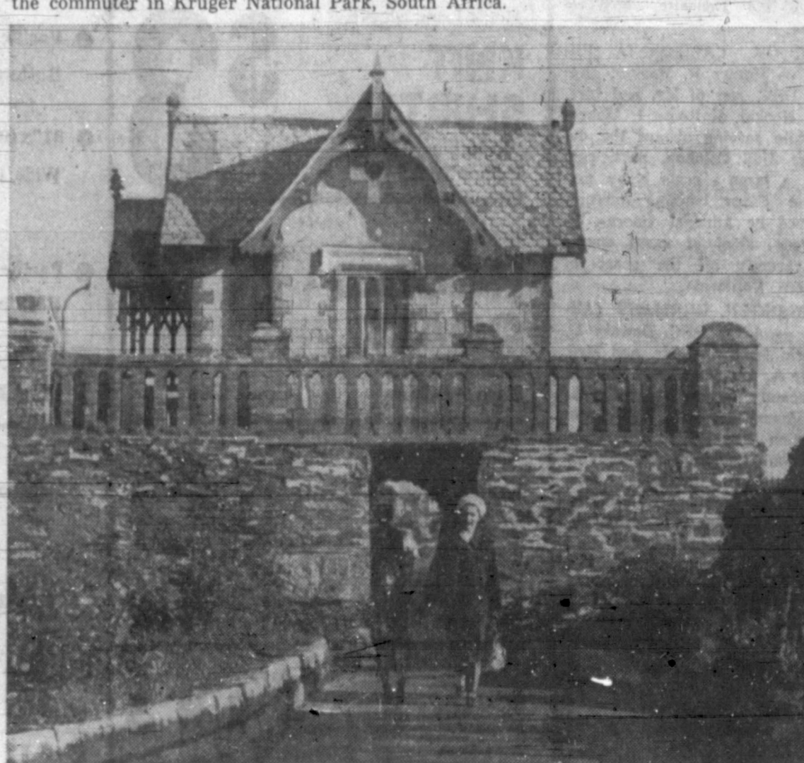
FIRM FOUNDATION —The foundation of this little doll's house was so good, a tunnel was cut through it for a sidewalk passage. Cliff Road sidewalk squeezes through under the tiny chapel at Gyllyngdune in Falmouth, England. The citizens want to renovate the famous structure, built by Rev. W. J. Coope, Rector of Falmouth from 1838 to 1870.
