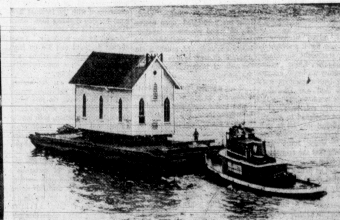
SHALL WE GATHER ON THE RIVER? —While it looks like the latest thing in river vessel drive-ins, the old St. John's Episcopal Church of Milwaukie, Ore., was being moved down the Willamette River to a new site at Oaks Historical Park by barge.
