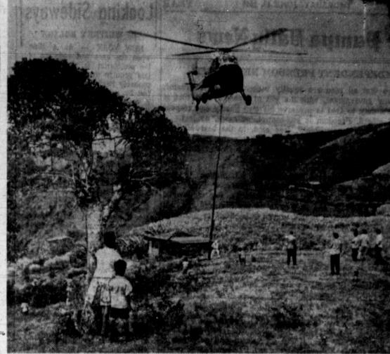
LIGHT WORK-Electricity comes to an isolated Puerto Rican home near San Juan as a helicopter lowers a power line pole into a hole. As local citizens of the rugged, mountainous country look on, a lineman guides the pole into placé.
