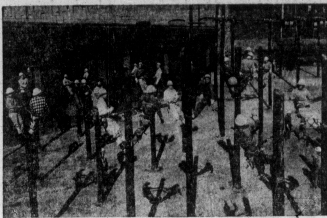
LOOK, MA, NO HANDS—Finding themselves up a tree is part of the daily routine of these linemen. They're playing "poleball," a form of training for electric utility linemen to get them used to hanging by straps around their waists. At Philadelphia Electric Co., these hangers-on are gaining confidence in themselves and their equipment. The ball is right of center in the photograph.
