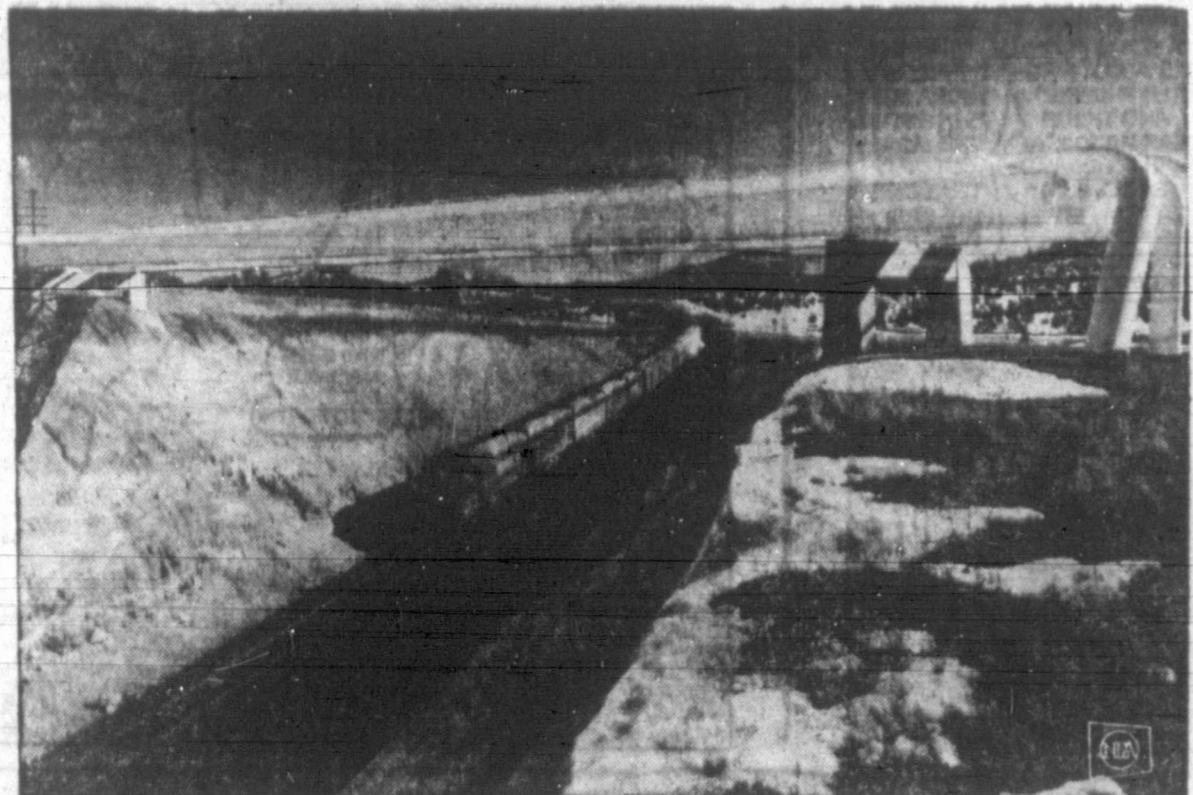
UNIQUE BRIDGE —What is said to be the only pipeline of its kind in the world soars 60 feet above main line tracks of the Santa Fe near Williams, Ariz. The bridge supports three pipelines of the El Paso Natural Gas Co. Going under the tracks at this point would have required cutting through some 40 feet of volcanic rock to construct a tunnel.
