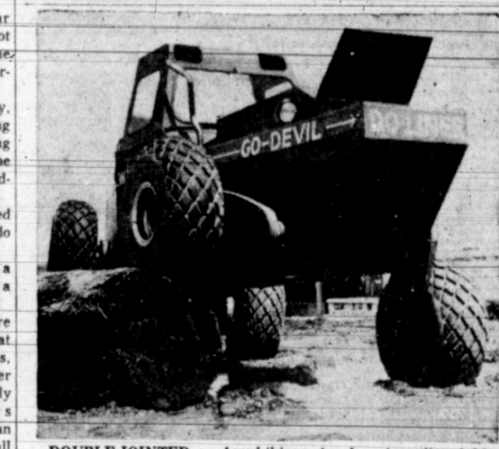
DOUBLE-JOINTED — Amphibious truck raises its right wheels to clear a big log in Portland, Ore., where the strange vehicle was invented by Elmer A. Wagner, a tractor manufacturer. Each of the wheels can be swung in a 360-degree arc. A propeller in rear drives it through water. Wagner says it can be used in the military, construction work, survey and exploration projects and hilly farming.
