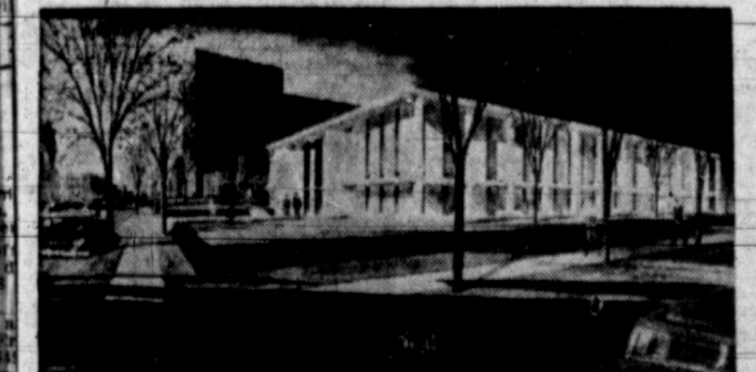
OPTIMIST HEADQUARTERS — Ground has been broken for the new Optimist International headquarters at St. Louis. The building, costing some $350,000 will house the 43 staff members of the organization's headquarters personnel. Construction of the building is expected to be completed in the near future.
