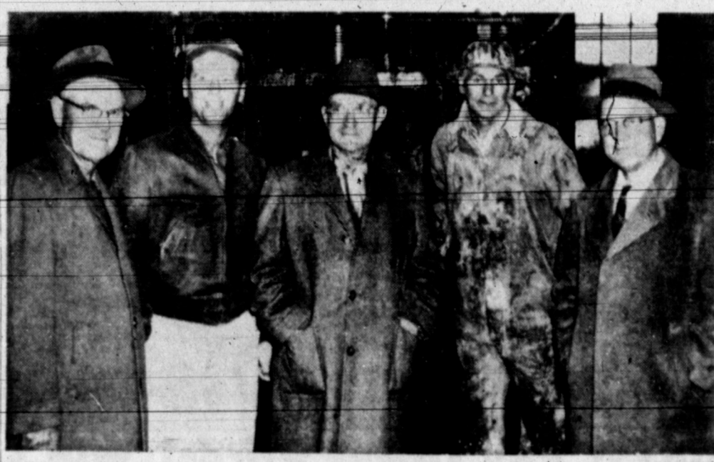
GETTING ACQUAINTED — Members of Chamber of Commerce Industrial Activities Committee, headed by Floyd Watson, yesterday visited the American-Marietta Company's pipe manufacturing plant located east of town at the site of the old Dancing refinery. The visit was a part of a schedule of calling on industries which have been located in Pampa in recent years. Shown above, left to right, are Floyd Imel, Floyd Crume, manager of the American-Marietta operation; Frank Culberson; Martin Nessman, pipe machine operator and Loyal Davies. (Daily News Photo)
