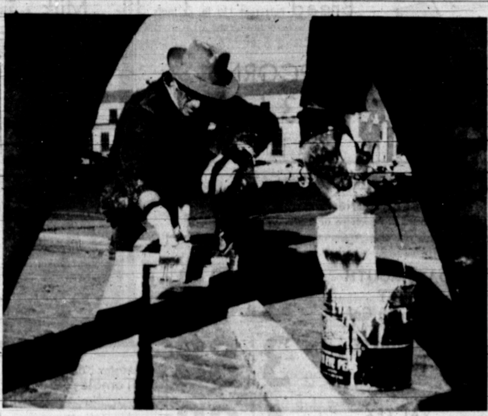
STREETS DRESSED UP — Pampa Street Department workers are at it again, repainting street division and safety lines through the city. This photograph was snapped on Cuyler looking north as O. Z. Kunkel was busily painting the crosswalk at Cuyler and Francis streets. The pair of legs that frame Kunkel are those of Jay C. Chennault. (Daily News Photo)
