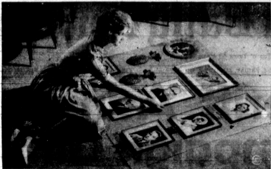
Preplan mounting of family portraits and wood plaques. Position first on brown wrapping paper and outline each piece. Paper can then serve as pattern for placing fasteners.
