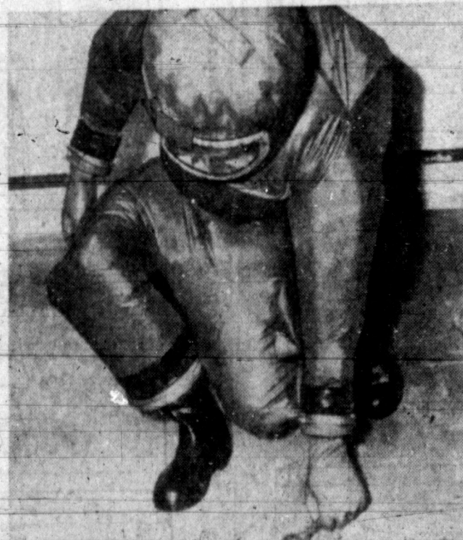
IT'S LIKE THIS —Testing the freedom of movement permitted by this new safety suit, rocket engine tester Austin Dickinson bends to pick up a wrench at Edwards Air Force Base, Calif. Moisture- and fireproof, the airtight suit, containing built-in breathing and cooling systems with a two-hour supply of liquid air, weighs about 25 pounds.
