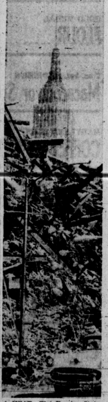
A HEAP —The Empire State Building is not buried in rubble despite appearances. Mountain of bricks and girders is all that remains of buildings in the Hill's Kitchen district. They've been razed to make way for a massive new co-operative housing project.
