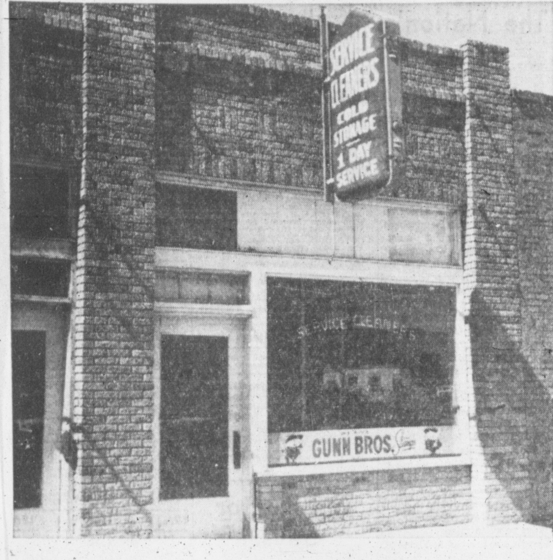
SERVICE CLEANERS — Oliver Jonas has been serving Pampa for 25 years in the dry cleaning business at 312 S. Cuyler. Service Cleaners features "Deodorized APCO-125" industrial cleaning solvent and Honeywell MagiCare automatic controls to assure the best in dry-cleaning at competitive prices.
