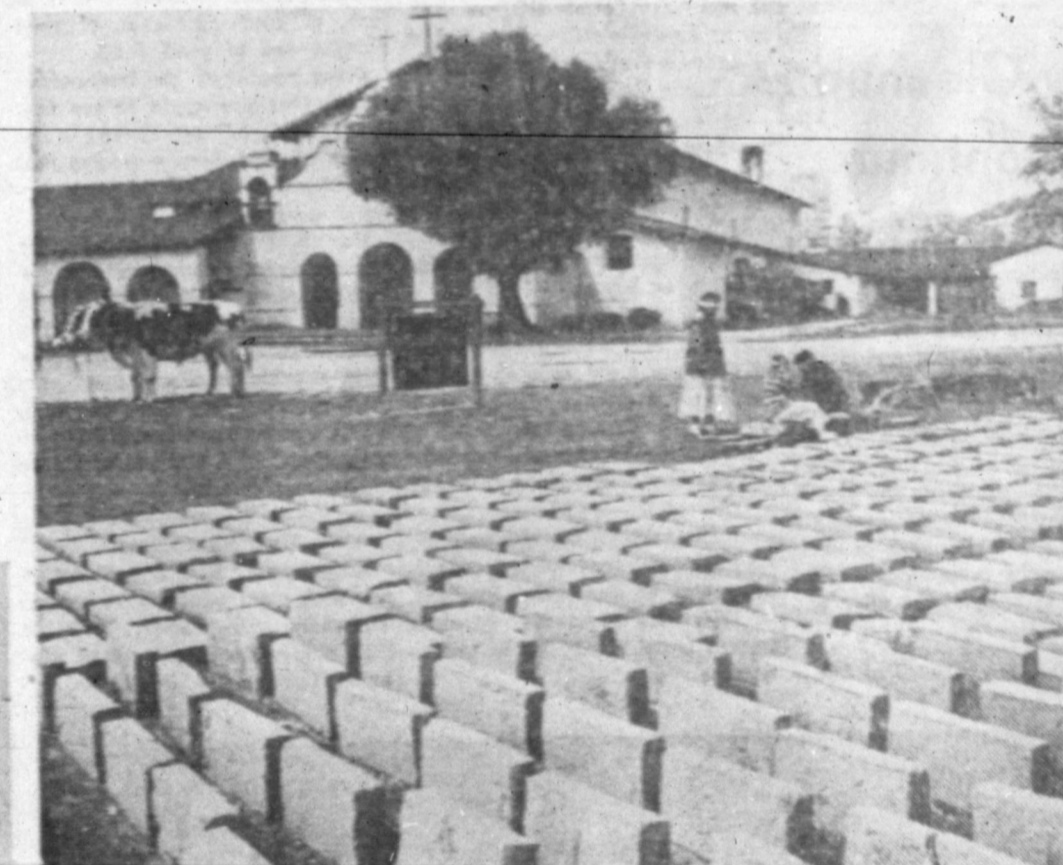
ADOBE ABODE —These adobe bricks were made in the ancient Indian way at Mission San Antonio, near Los Angeles, Calif. They're spread in the sun to dry, a process that takes three days. During that time, they must be turned often to "cook" evenly. Used to build the mission in the background in 1771, the bricks are made of adobe soil, straw and water. Each finished brick weighs about 60 pounds.
