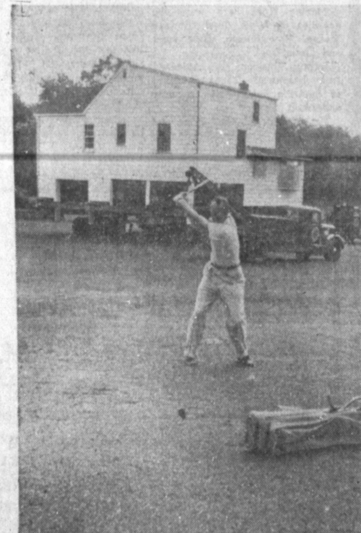
A HOUSE IS NOT A HOLE —Okay, so there's a house rolling down the fairway. But it takes more than a mere house-in-the-way to disconcert this intent golfer who's concentrating on his tee shot at the Englewood, N. J., golf course. Uprooted to make room for a new highway, the house was being towed across the links to its new location. It never was really in anyone's way on the links.
