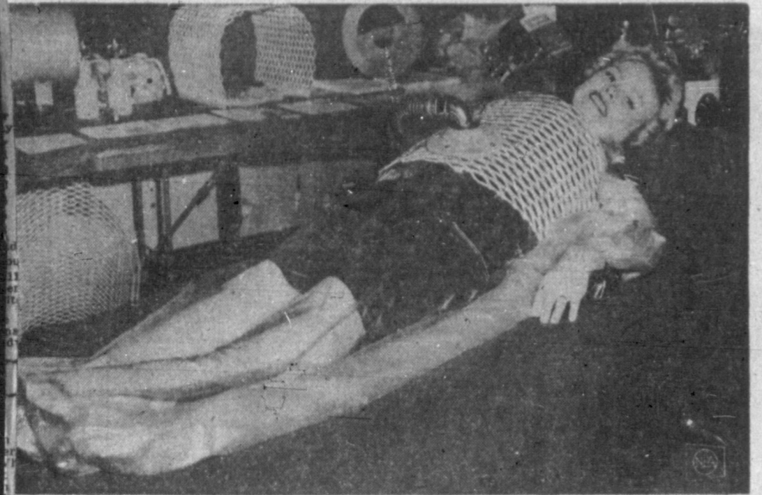
RAINCOAT RESPIRATOR—Gail Andrews models a plastic bag respirator in Chicago. Using a modified vacuum cleaner motor, the bag fits like a big raincoat. Device does the breathing for the patient in polio and some surgery cases. It was invented by John H. Emerson of Cambridge, Mass.
