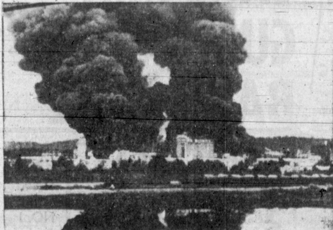
EXPLOSION KILLS ELEVEN — Hit by an explosion, the Tennessee Eastman Co. in Kingsport, Tenn., burns out of control hours after the blast. Eleven persons were killed in the explosion.
