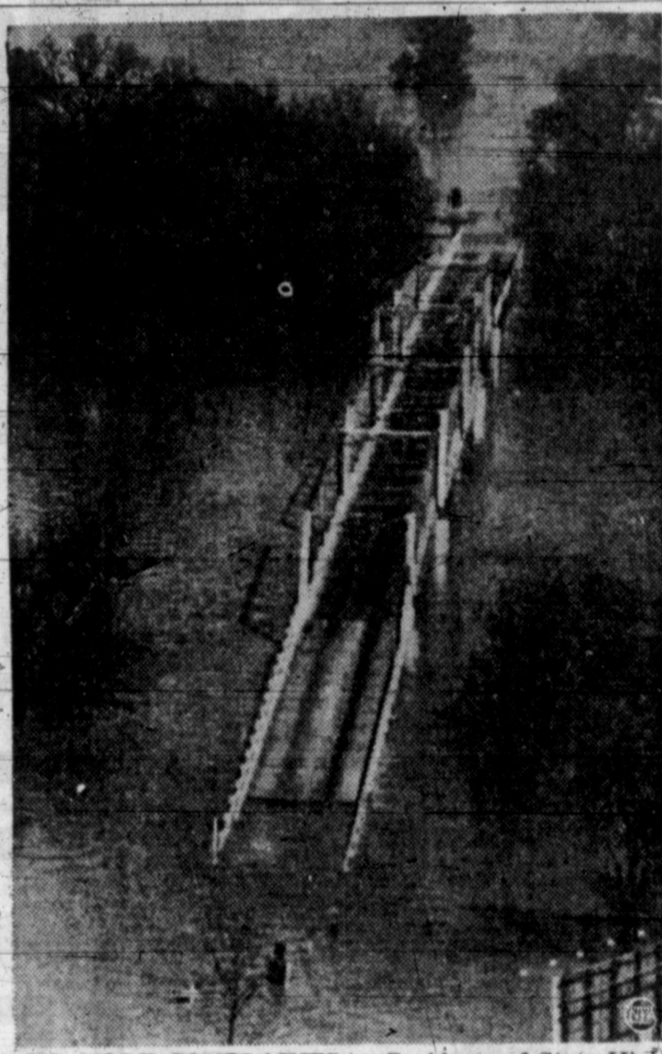
NO MORE COMPLAINTS — Residents of State Highway 143 complained when authorities closed the Tyler-Goodwyn Bridge over the Alabama River north of Montgomery. But there have been no more complaints since the flooding river crested and almost covered the bridge. (NEA Telephoto)
