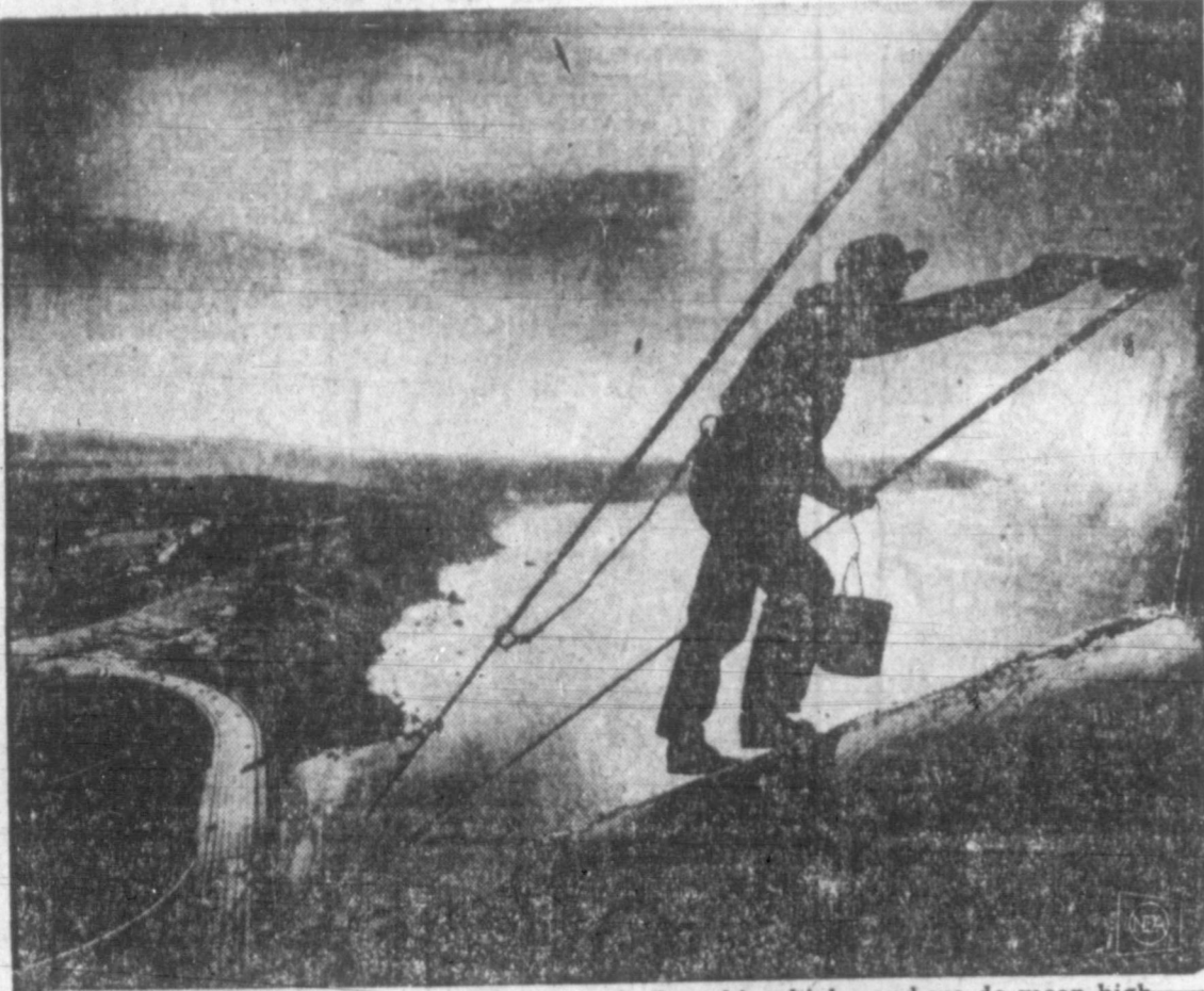
PICTURE PUZZLE —You see painter Jerry Cuff working high—and we do mean high—on the Golden Gate bridge at San Francisco. Question: From where did the photographer make the picture? He was on a girder close by, holding camera on an extension and tripping it with a long cable release. In background is a sweeping view of western San Francisco.
