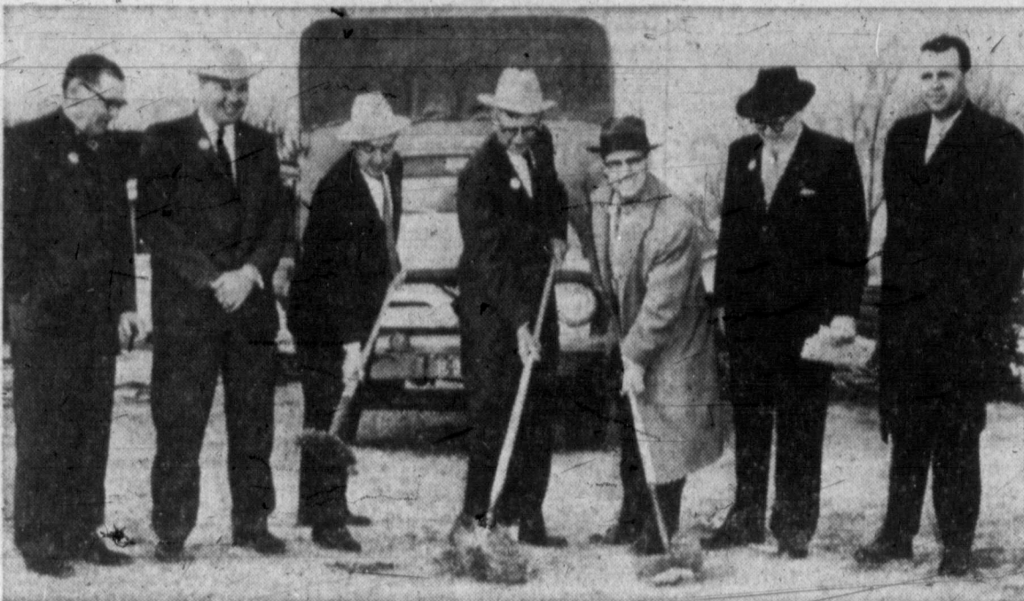
GROUND IS BROKEN — This was the scene Monday when the first earth was turned at the site of the new home of the Soft Water Service Co., 314 S. Starkweather. Left to right in the photo are E. O. Wedgeworth, manager; Allen Ritter, contractor for the new building; James B. Massa, co-owner of the company; County Clerk Charles Taut, the firm's first customer; John L. Rankin, co-owner; William J. Smith, company attorney; and E. Roy Smith, chamber of commerce president.
