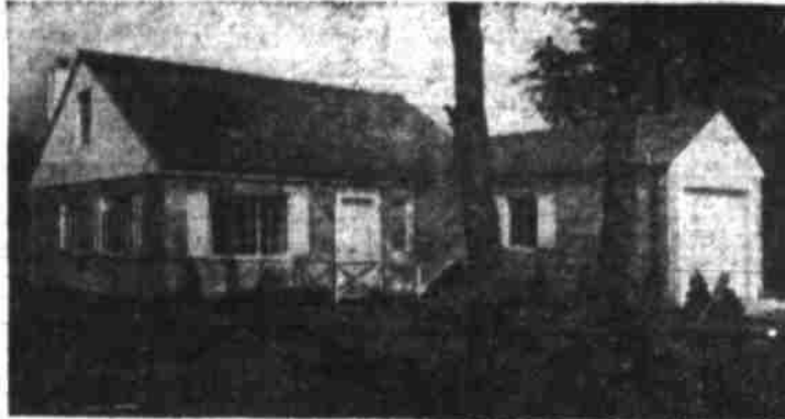
POURED IN A MOLD , with walls insulated, this concrete house is Patrick J. Callan's answer to slow building methods. Living room form at right weighs five tons.
