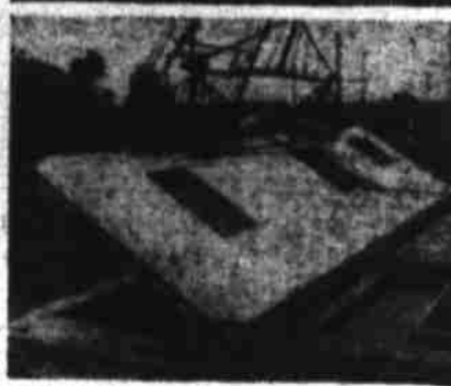
POURED on the ground , Myer's walls are tilted in place.
