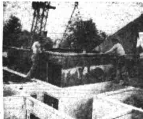
POURED IN A MOLD , with walls insulated, this concrete house is Patrick J. Callan's answer to slow building methods. Living room form at right weighs five tons.
