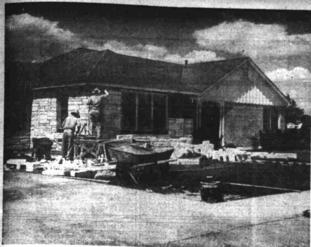
AUSTIN STONE , gaining in popularity all the time, is blended with brick in this home enlargement. (Photos by Jack M. Haynes)
