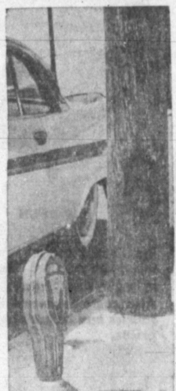
SINKER—This Memphis, Tenn., parking meter isn't designed for small foreign cars. Improperly anchored in the cement, the meter sank into the soft earth of its own weight.
