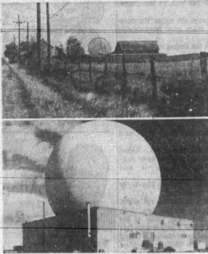
HERE'S WHY —The oversized ball this golfer is about to whack is really not a golf ball at all (left). It's a 15-story Ballistic Missile Early Warning System radome, housing a tracking radar antenna and pedestal at the Radio Corporation of America's engineering test facility at Moorestown, N. J. Another photo of it is shown at upper right and, below, a closeup. Other BMEWS sites are at Thule, Greenland, and Clear, Alaska.
