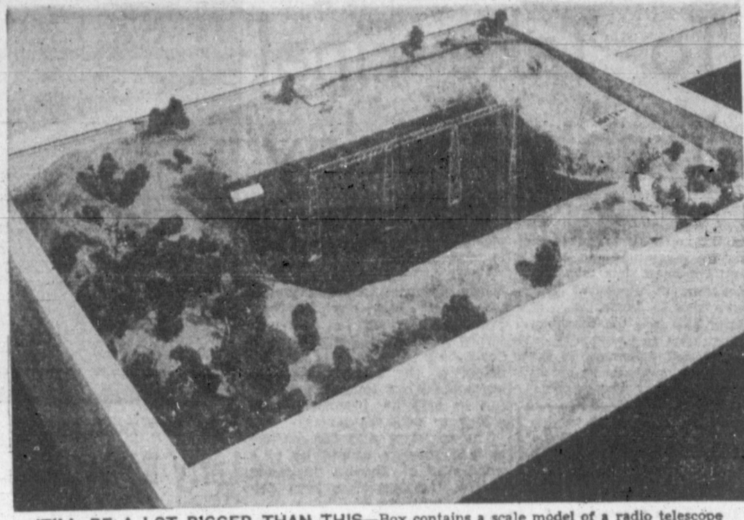
IT'LL BE A LOT BIGGER THAN THIS—Box contains a scale model of a radio telescope which will be the biggest in the world when it's built this fall in Danville, Ill. The University of Illinois will construct and operate the telescope under the sponsorship of the Office of Naval Research. The telescope will cover a 5½-acre natural valley. Its 160,000 square feet of receiving area will be covered with an asphalt liner and a wire-mesh reflecting surface. Four wooden towers 165 feet tall will carry 300 feed elements to the big "ear."
