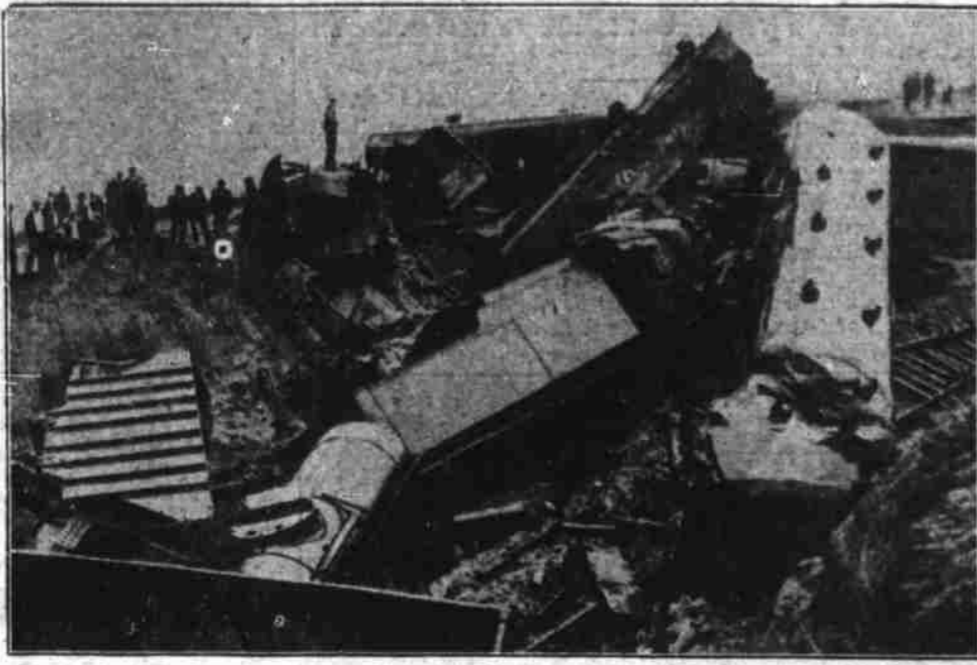
The engineer and fireman of a passenger train were killed near Fredericksburg, Va., when that train collided with a freight train. This picture provides a general view of the wreckage which resulted. (Associated Press Photo)
