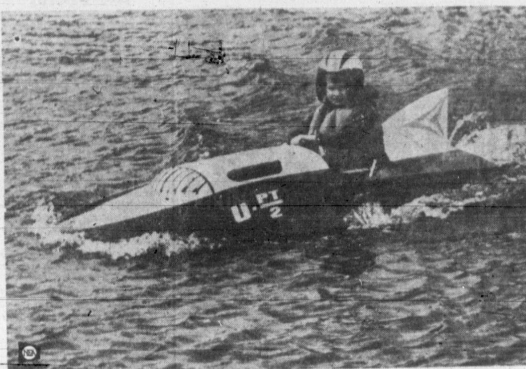
**CAPTAIN KID**—Kallen Moll, 5½, skips her hydroplane, U.P. T/2, which translates as Half Pint, on Lake Washington in Seattle. Her dad, John Moll, built the 85-pound, plywood-hull craft powered with a 3½-horsepower chain-saw engine. Wee captain was off and running.
