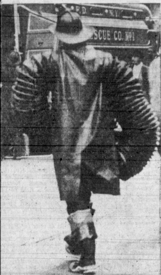
CORDION-ARMED—New York City firemen don't come equipped with strange coat sleeves like these. The odd embellishments are collapsible air ducts, used to pump air to firemen working in smoke. They were used in a subway blaze.
