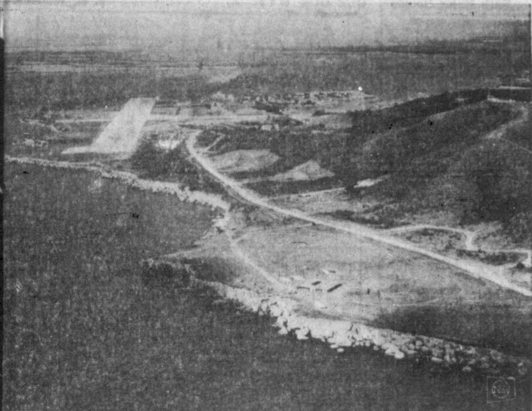
GUANTANAMO is a 45-square-mile, 76 million dollar installation. Photo, above, shows two air strips—able to handle jets—crisscrossing at edge of Guantánamo Bay. Six thousand men guard Gito. Thousands more are near, aboard ships always in area. Some 3,500 Cubans, many pro-Castro, help service the base and pose threat of sabotage. Cuba furnishes power and water but the base has auxiliary means and supplies. Armament, air and naval power weigh heavily in U.S. favor against a possible overt move by Castro.
