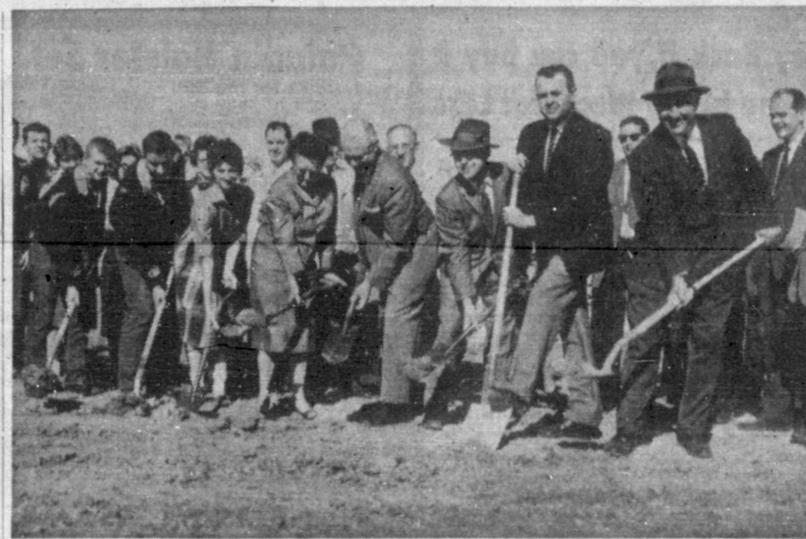
SHOVEL WELDERS — Starting off the construction of Pampa's long-sought youth center yesterday in ground breaking ceremonies at the site between Harvester and Kentucky streets, are left to right, and using the shovels, Lucky Dunham, president of the high school student body; Bill Nslaga and Sue Guthrie, of the student council; Mrs. Inez Carter, strong financial supporter of the center; Dr. Joe Donaldson, center president; City Manager John Kooztz; E. Roy Smith, president of the Pampa Chamber of Commerce, and Fred Neslage, vice-president of the center, and the Rev. Richard Crews, at Neslage's left, who gave the invocation. (Smith Studio Photo)
