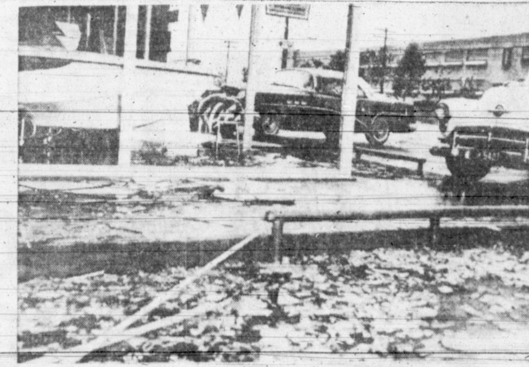
HAIL DAMAGE — Hail up to the size of baseballs shattered plate glass windows and roofs in San Angelo, Tex., causing damage estimated at between two and three million dollars.
