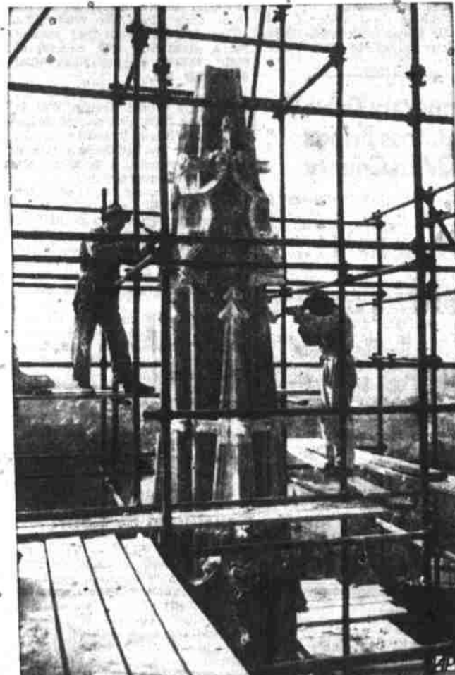
REPAIR DAMAGE OF TIME —Stonemasons work on spire of Cathedral of St. Pierre, Beauvais, France, to repair Gothic architecture which has suffered from time and weather.
