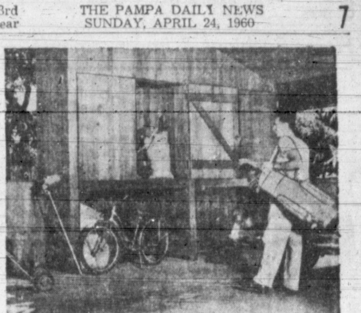
CARPORT WALL provides handy built-in storage space for gardening tools, gear, fertilizer, seeds and pots. There is even a special compartment for bikes in this well planned wall.
