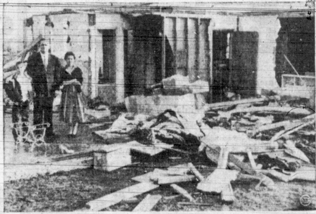
HOME DESTROYED — The Rev. Murlie Rogers, pastor of the Sunnyside Baptist Church, his wife and their son stand in the wreckage of their home destroyed by a tornado that ripped into Sunnyside, Tex., and killed three persons and injured many others. Rev. Rogers was inside the house when the twister struck, moving the house some 100 feet off its foundation. The pastor received some cuts, but was not seriously injured.
