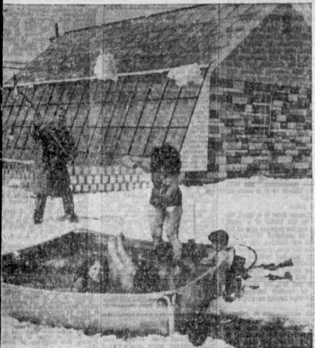
SUNNY SIDE OF THE HOUSE —That is no greenhouse, above, which the Harry T. Thomason family lives in. The glass covers a solar heating plant on the side of the three-bedroom District Heights, Md., house. It enabled Thomason to heat his home this winter with energy from the sun and 15 gallons of fuel oil burned in a standard furnace. To demonstrate, Mrs. Thomason and the kids cavort in an outdoor pool filled with water also warmed in the solar unit. Daddy livers up the party with a little unsolicited snow.
