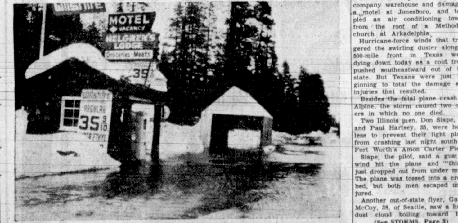
HIGHWAY COVERED —Considerable damage has been reported from areas where flood-swollen rivers left their banks after two days of heavy rains in California. Here, flood waters of the Yuba River flow over Highway 40 about a quarter of a mile from the Rainbow Inn at Squaw Valley, site of the upcoming Winter Olympics.
