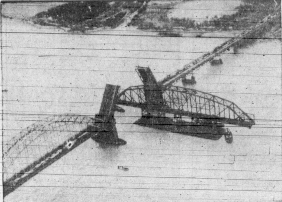
IT FINALLY HAPPENED—Ever wait at a drawbridge while another bridge went by? Amazed motorists waiting to cross the Tacony-Palmira Bridge linking New Jersey and Pennsylvania saw a 533-foot bridge go. The bridge was moved down the Delaware River.
