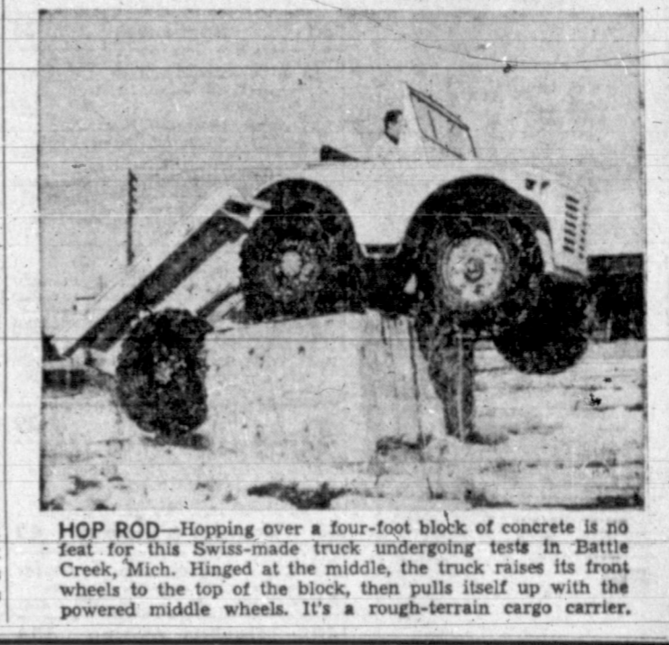
HOP ROD—Hopping over a four-foot block of concrete is no feat for this Swiss-made truck undergoing tests in Battle Creek, Mich. Hinged at the middle, the truck raises its front wheels to the top of the block, then pulls itself up with the powered middle wheels. It's a rough-terrain cargo carrier.
