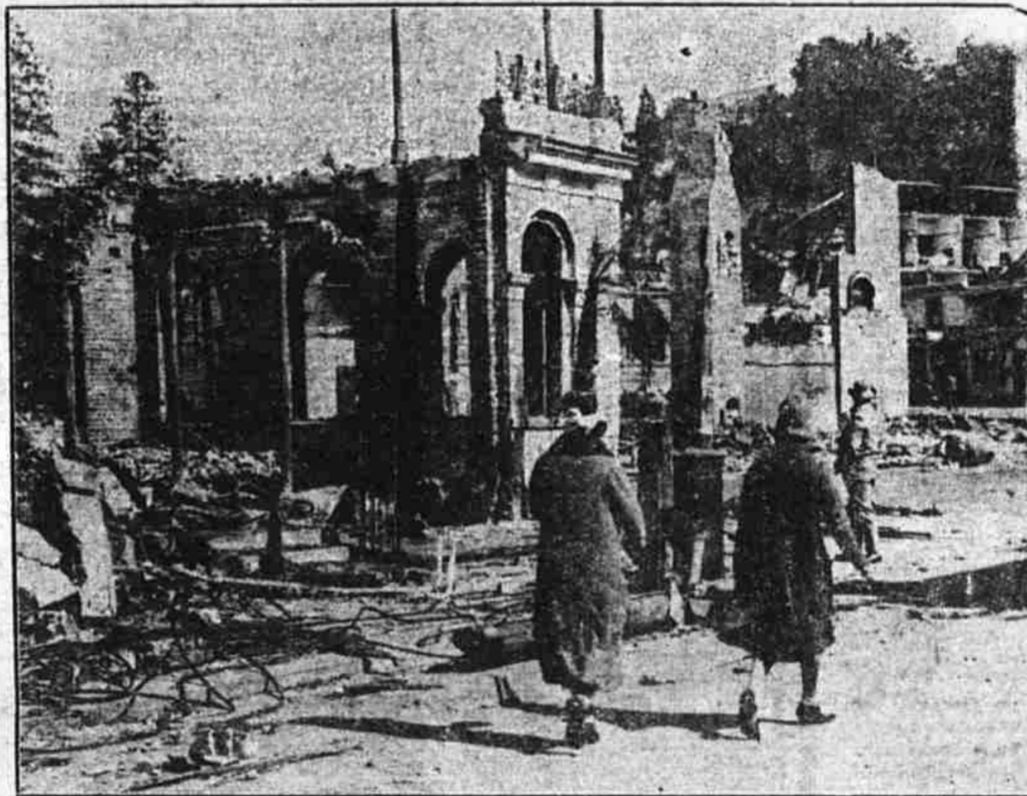
Only slender columns of stone and mortar were left standing in the section of Napier, New Zealand, shown here, following a series of earthquakes that rocked North Island. Residents are shown surveying the damage done by the quakes which killed more than 200 and injured 1,500.
