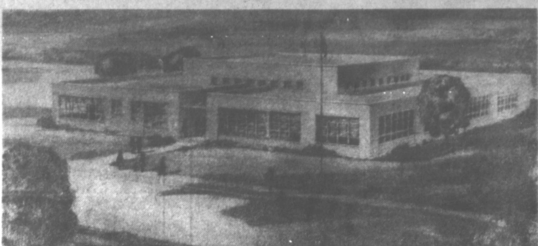
NEGRO SCHOOL —This building planned for Negro students in the overall expansion designs for increasing teaching facilities in the Pampa schools will contain an auditorium-gymnasium, four elementary class rooms, two high school class rooms, a homemaking lab, industrial shops, and a library, in addition to the administrative offices. The crowded conditions in Pampa schools that have developed within recent years are particularly bad in the Negro school, Superintendent Knox Kinard said recently.
