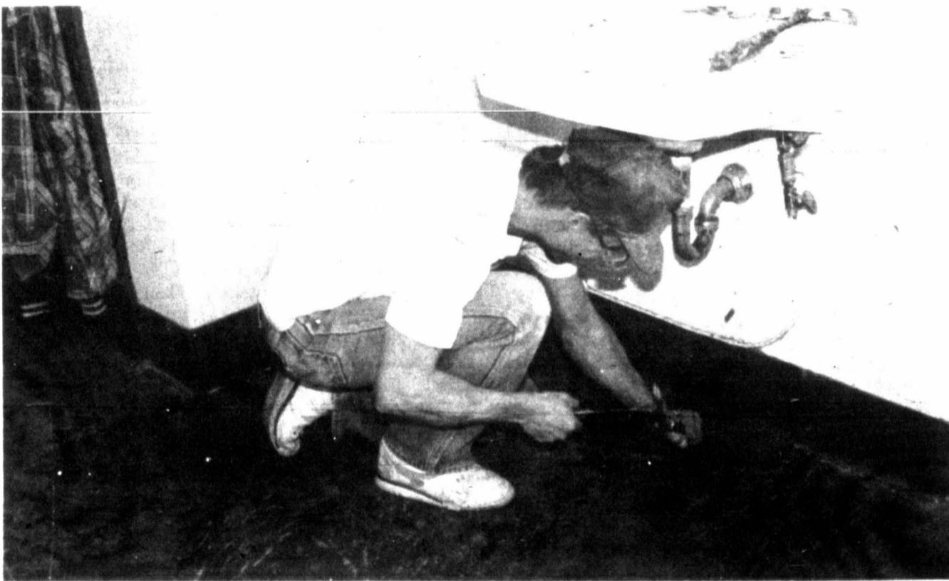
Mike Knutson of Hardy Knutson Masonary Contractor scrapes tile Thursday off the floor of the women's restroom on the third floor of the Gray County Courthouse in preparation for the placing of new tile.
